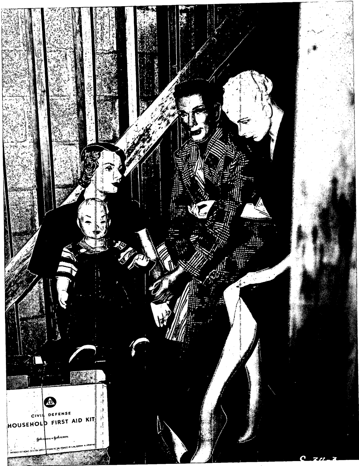
Fig. 9—Basement corner room (at 7500 ft) after blast.
